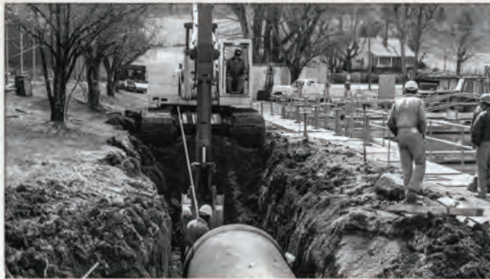
LEFT: Workers install new pipe at the Roy Oakes Filter Plant in the 1970s.
